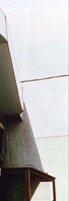
FIGURE 2. Hoods that cannot be designed with total enclosure should be located as close to the source as possible. A side draft hood located twice the distance from the source can require as much as four times the exhaust volumetric flowrate
