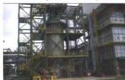
The largest radiometric imaging system for safety monitoring of a petrochemical processing vessel uses 14 Mikron infrared cameras and MikroSpec R/T software. It has been online for more than a year monitoring this Chevron-Texaco-designed gas separation system in Texas.
